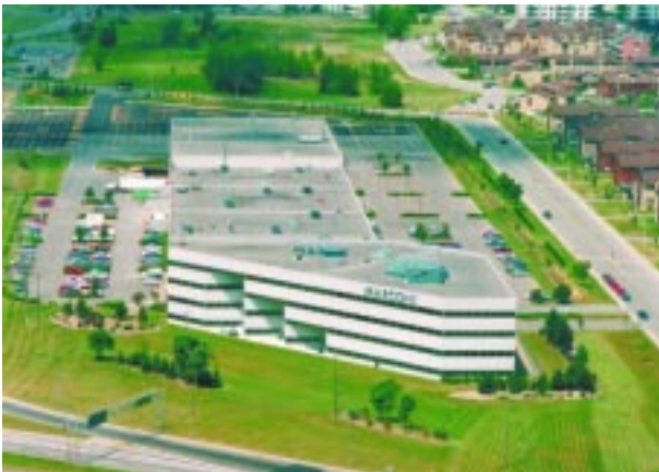
1 The headquarters of Marconi Canada
